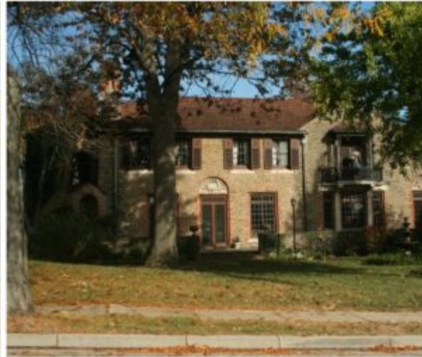
Photo 2. 960 Avondale Avenue (1912), Harry L. Linch House, Grosvenor Park, Renaissance.
