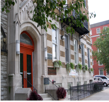
Emanuel Community Center, photo by Chris Hill, 2014
