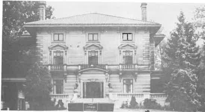
Conversion of a large old single family home to institution while preserving the original physical character of the structure.
