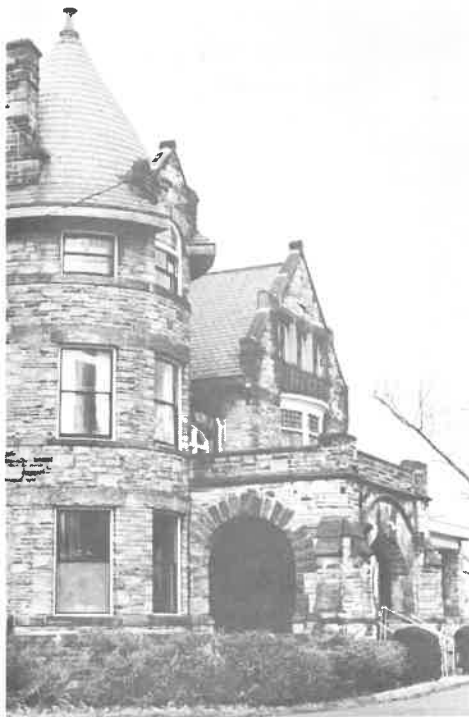
Robert Mitchell's 84 year old mansion, a community landmark and historic monument, is being utilized for educational purposes and is in need of rehabilitation.
