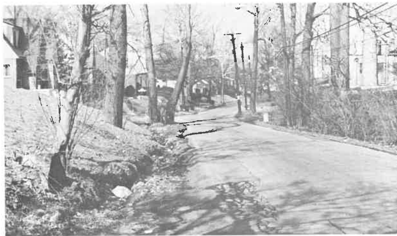
Street conditions in some arteries are deteriorated and the lack of curbs and sidewalks is creating pedestrian and vehicular problems.
